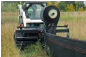
Silt Fence Installer P. 102
